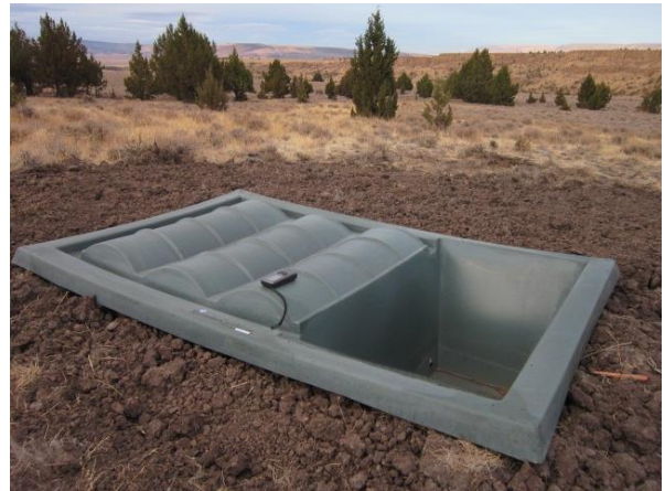
500-gallon guzzler installed in Palomas, NM.
