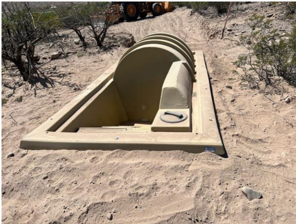
1000-gallon guzzler installed in Engle, NM.
